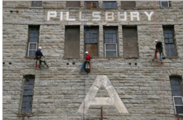
Dan Gach, Paul Whitenack, and Lucas Malm of Wiss, Janney, Elstner Associates' "difficult access team" test the exterior of the Pillsbury A-Mill last year in Minneapolis. The activity is one of the measures engineers and architects take to make sure older buildings can be used for new purposes. (SUBMITTED PHOTO: WISS, JANNEY, ELSTNER ASSOCIATES)
